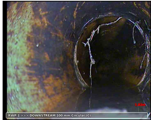
20191023-085610-snap0005.jpg, 00:01:21, 1.82 m Roots, fine at joint
