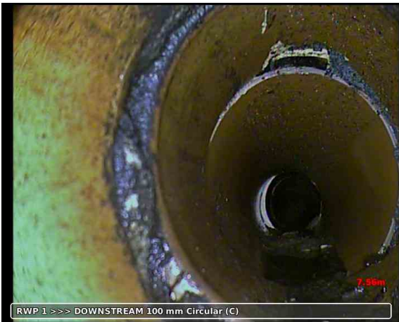
20191023-085610-snap0014.jpg, 00:04:29, 7.56 m Hole in drain or sewer, at 12 o'clock
