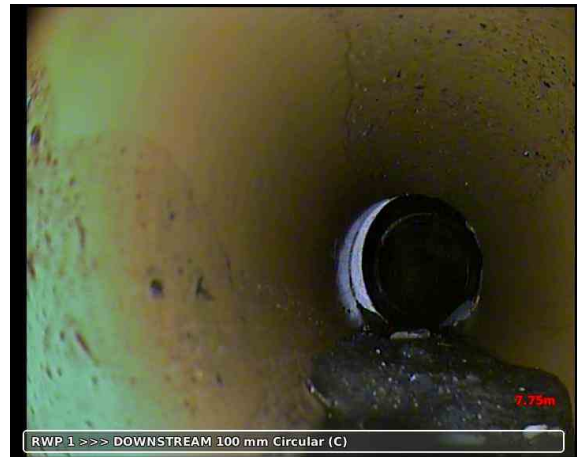
20191023-085610-snap0015.jpg, 00:04:50, 7.75 m Settled deposits, fine, 10% % cross-sectional area loss
