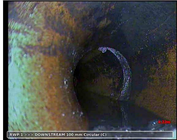
20191023-085610-snap0009.jpg, 00:02:37, 4.22 m Line deviates left, 30
