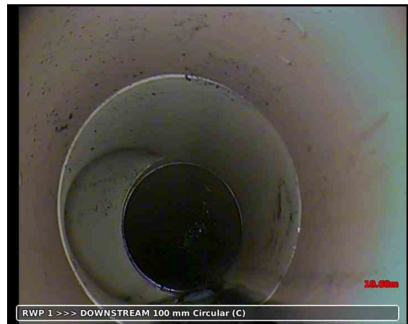
20191023-085610-snap0023.jpg, 00:07:49, 10.60 m Finish node type, other special chamber, reference number: DOWNSTREAM, NEW PVC
