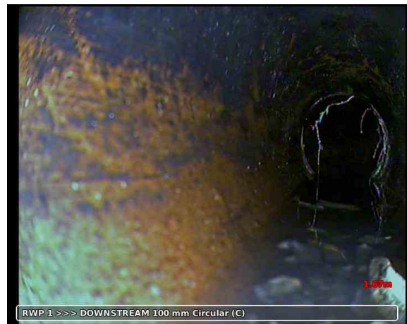
20191023-085610-snap0003.jpg, 00:01:05, 1.67 m Material changes to vitrified clay, CHANGE V.CLAY
