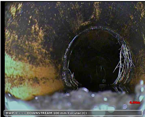
20191023-085610-snap0010.jpg, 00:03:00, 4.94 m Roots, tap at joint
