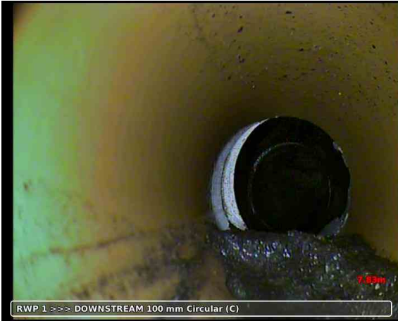
20191023-085610-snap0016.jpg, 00:05:17, 7.83 m Material changes to polyvinyl chloride
