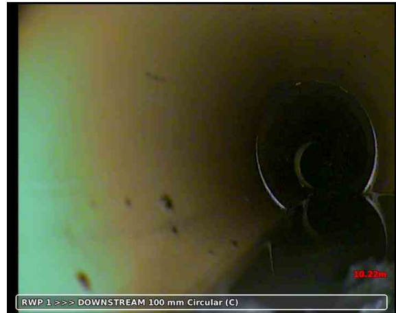
20191023-085610-snap0020.jpg, 00:06:42, 10.22 m Water level, 15% % of the vertical dimension
