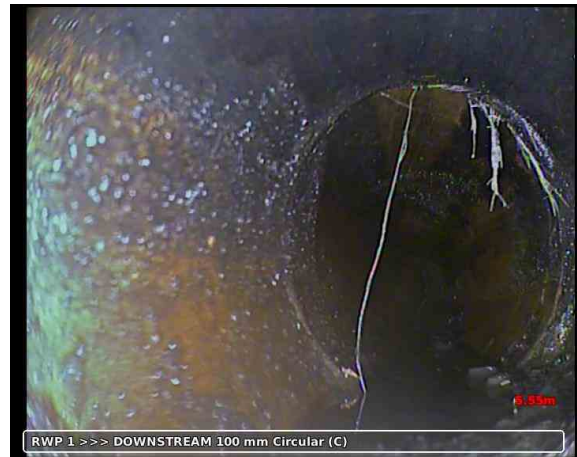
20191023-085610-snap0011.jpg, 00:03:25, 5.55 m Roots, fine at joint
