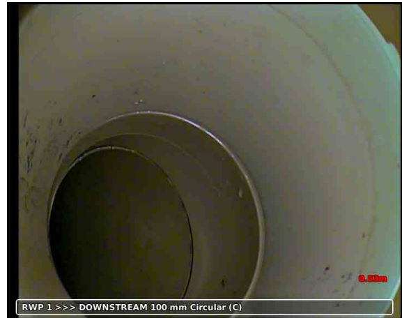
20191023-085610-snap0001.jpg, 00:00:38, 0.53 m Line deviates left, 30
