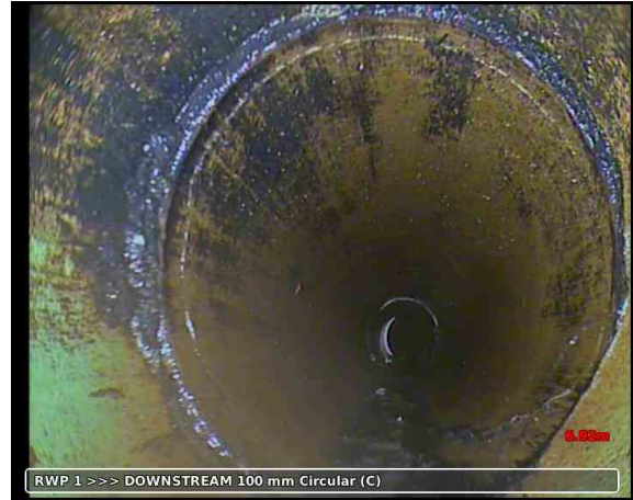
20191023-085610-snap0013.jpg, 00:03:55, 6.92 m Crack, circumferential, from 07 to 05 o'clock
