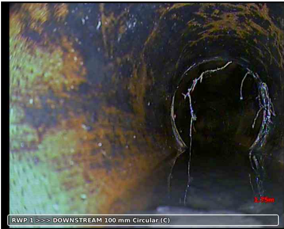
20191023-085610-snap0004.jpg, 00:01:14, 1.75 m Water level, 10% % of the vertical dimension
