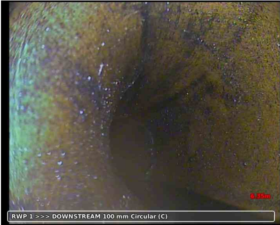
20191023-085610-snap0012.jpg, 00:03:39, 6.35 m Line deviates left, 30
