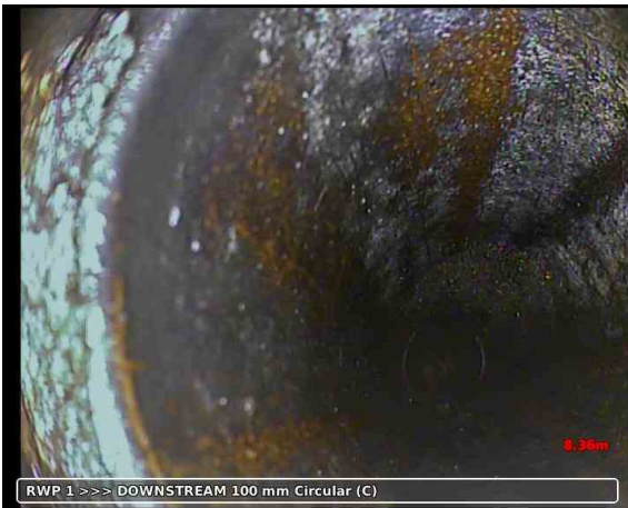
20191023-085610-snap0018.jpg, 00:05:58, 8.36 m Material changes to vitrified clay
