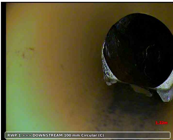
20191023-085610-snap0002.jpg, 00:00:53, 1.22 m Joint displaced, medium
