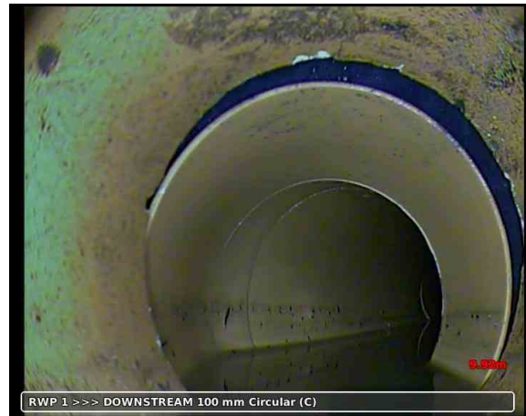
20191023-085610-snap0019.jpg, 00:06:30, 9.92 m Line deviates right, 15
