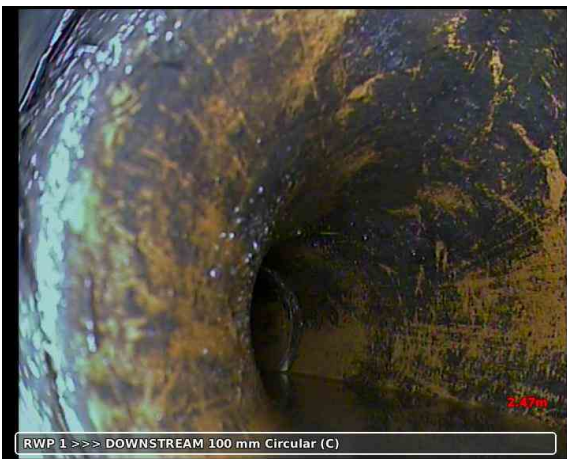
20191023-085610-snap0006.jpg, 00:01:39, 2.47 m Line deviates left, 30
