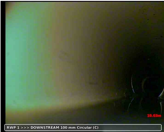
20191023-085610-snap0021.jpg, 00:07:17, 10.03 m Material changes to polyvinyl chloride
